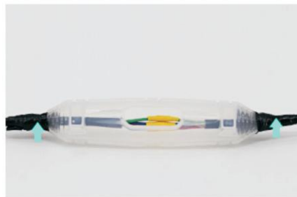
5. Stretch the insulating self-adhesive tape by 2-2.5 times at both ends of the plastic shell.
