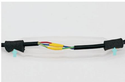
4. Wrap the rubber foaming strip around the two ends of the cable.
