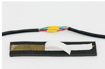
2. Remove the double-sided tape from the rubber foaming strip.
